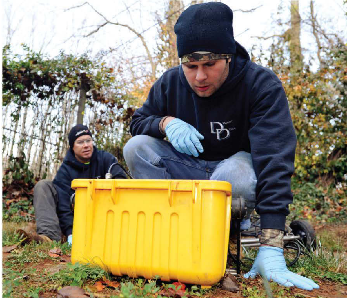
Nick Santoni looks at a camera image on a monitor while Wes Fogelman feeds the camera through a drain line.
